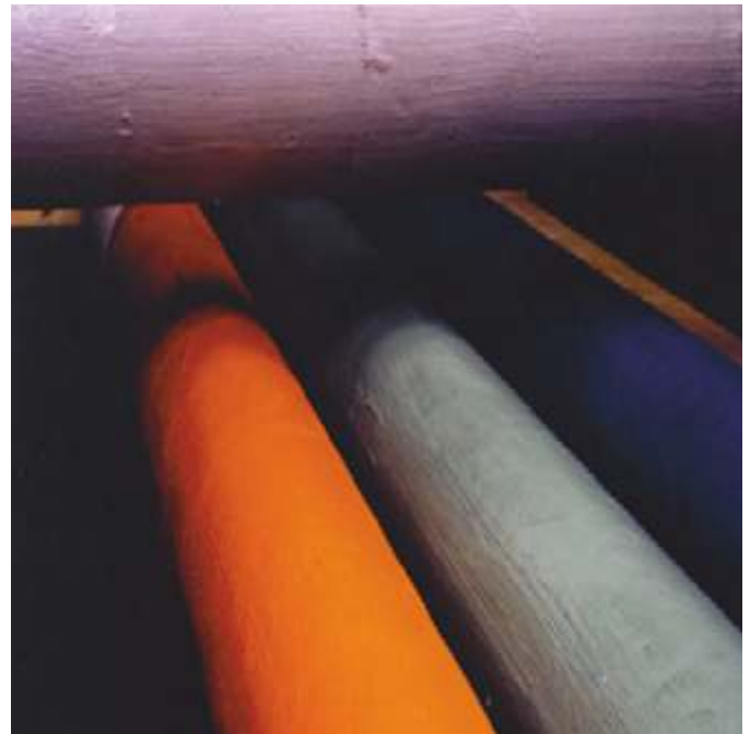
TIKI KCP9 applied in 2 application with reinforcement mesh in between. Supplied in two colors to differentiate between each layer.
